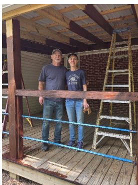
Doug and Patty Cooke staining a covered deck.
