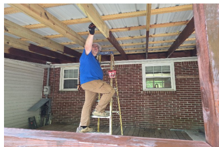
Scott Monday staining the rafters.
