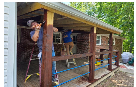
Doug Cooke and Scott Monday staining a covered deck.
